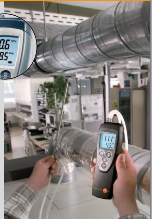
Measuring process air
